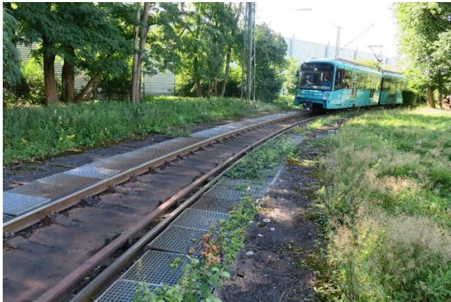
Figure 8: Light rail vehicle at the exit from the south-eastern track bend. Photo by A. Schäfer/FCP IBU
